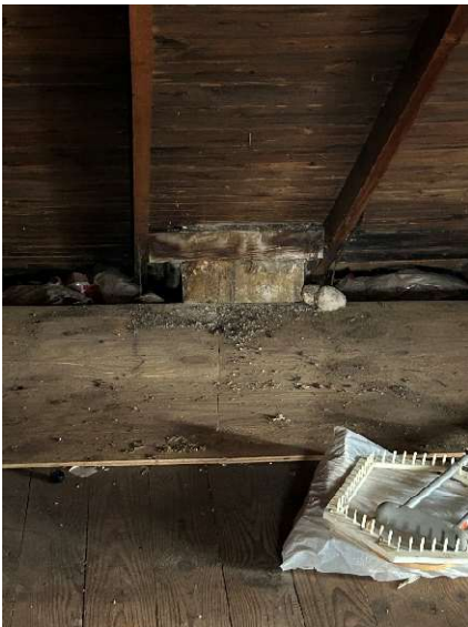
Masonry around the chimney in the attic
